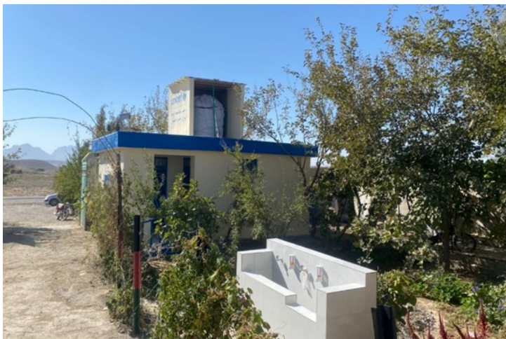
Figure 4. Construction of safe water facility in a health care center, Zabol province, Afghanistan, Oct 2022
