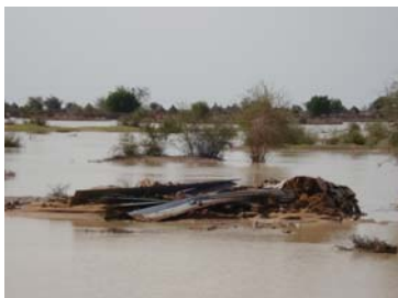
House destroyed by floods in Al Hireiza, North Kordofan
