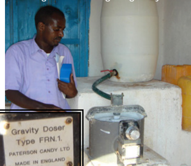
The Junction: chlorination of Berbera drinking water through a gravity doser
