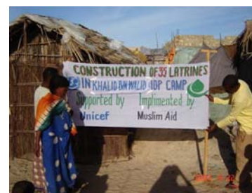
Muslim Aid constructed 35 latrines at Khalid bin Walid IDP camp in Kismayo with support from UNICEF
