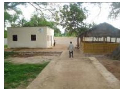
The new Janale MCH constructed by COSV with support from WHO
