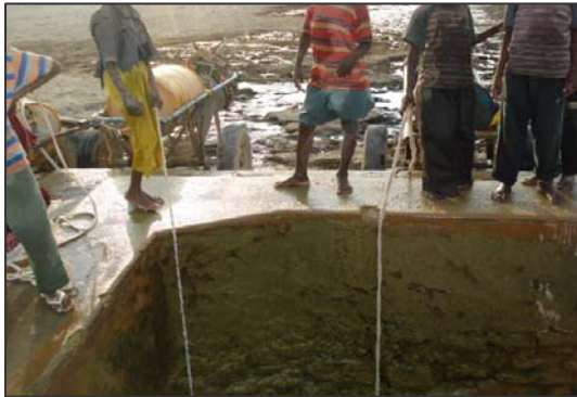
Well in Rabdhure District: Visible garbage in well and poor drainage
