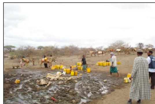
A sand basin originally created for water catchment in Washago with no adequate drainage and posing risk of communicable disease
