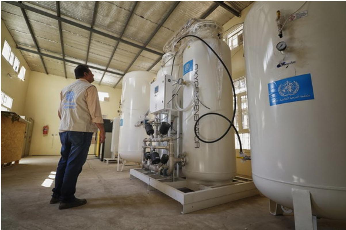
Each oxygen station has the capacity to fill 200 oxygen cylinders per day, helping to fill the gap of the inpatient and intensive care units in Al Thawra Hospital
