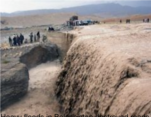
Heavy floods in Balochistan destroyed roads and bridges
