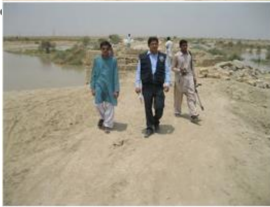
Surveying the damage to
