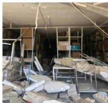
Heavily damaged central drug warehouse, WHO Lebanon
