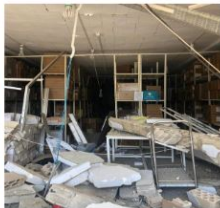
Heavily damaged central drug warehouse, WHO Lebanon
