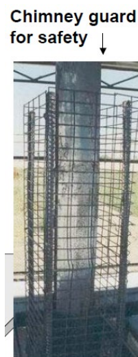
Fig. 10. Chimney with protected fence
