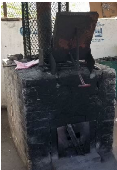
Hodeidah De Montfort incinerator Photo 6.
