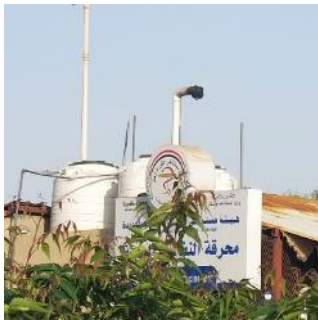
Roof plastic tanks in Hodeidah
