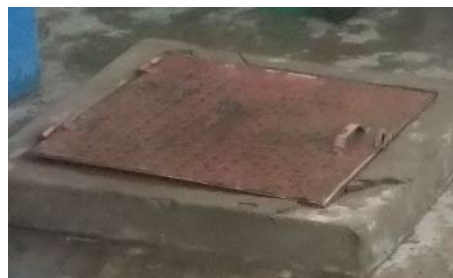
Non-corroded iron covers in Sa’adah
