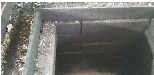
Hodeidah De Montforte incinerator
