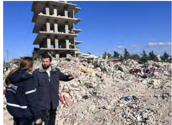
Infrastructure damages in Latakia due to the earthquake
