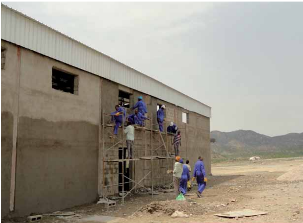
● Construction of a new slaughterhouse, Borama, Somaliland
