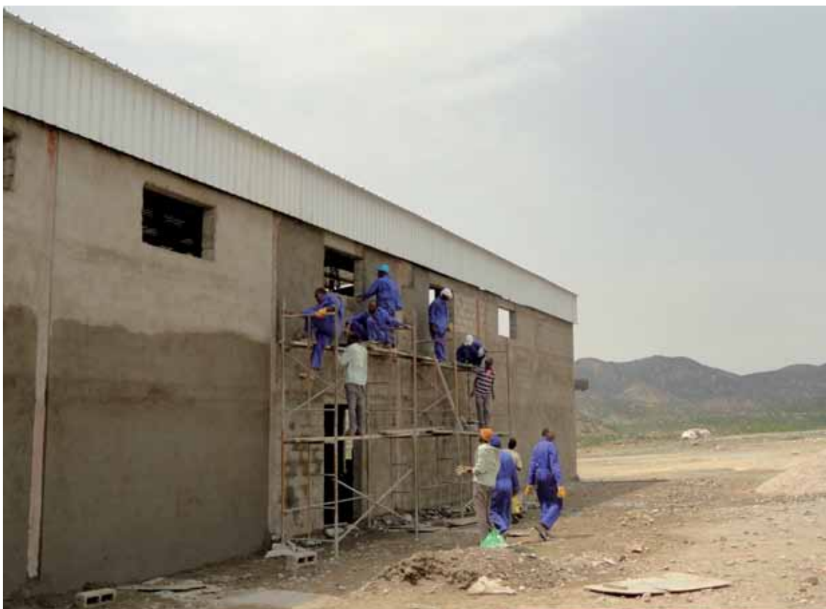
● Construction of a new slaughterhouse, Borama, Somaliland
