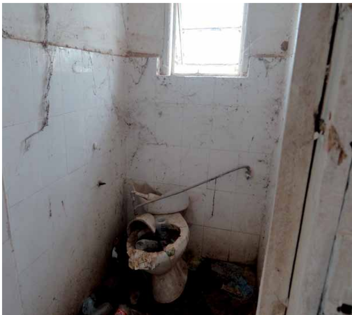
● Toilet facilities in Hargeisa General Hospital, Hargeisa, Somaliland
