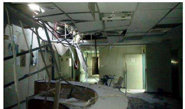
The Jordanian field hospital damaged on November 19. (photo by Mahmoud Halabi – WHO).
