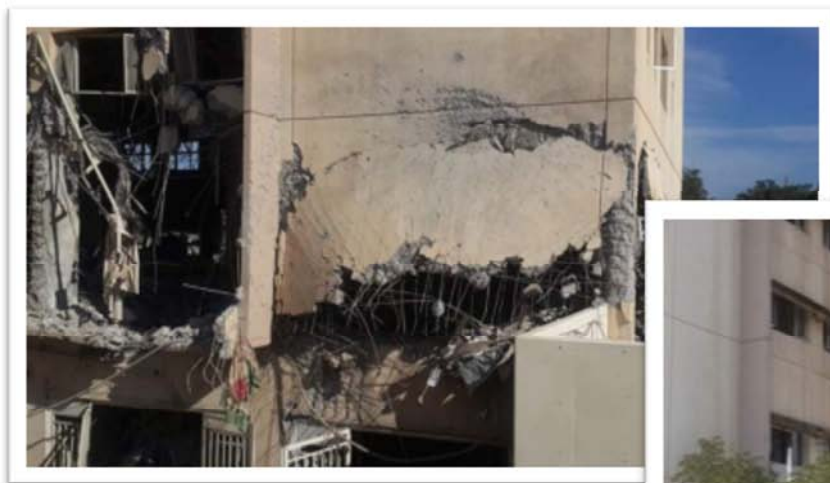
A severely damaged Al-Ramadi General Hospital
