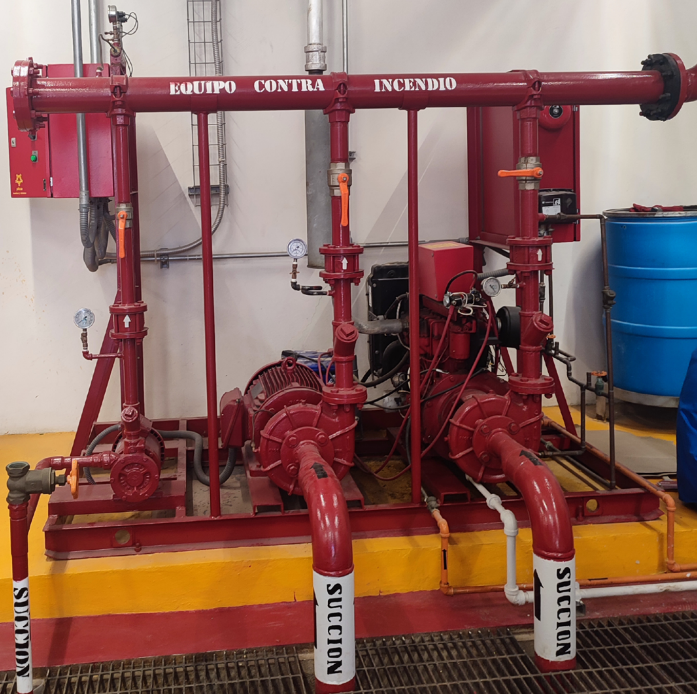
■ Redundancy of a firefighting system. Hospital General Regional 2, IMSS, El Marqués, Querétaro, Mexico. WHO Collaborating Centre MEX-35 for Resilient Health Services. 2021
