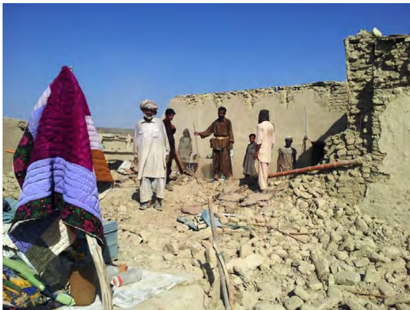
damages after earthquake in Awaran town on 24 th Sep-2013
