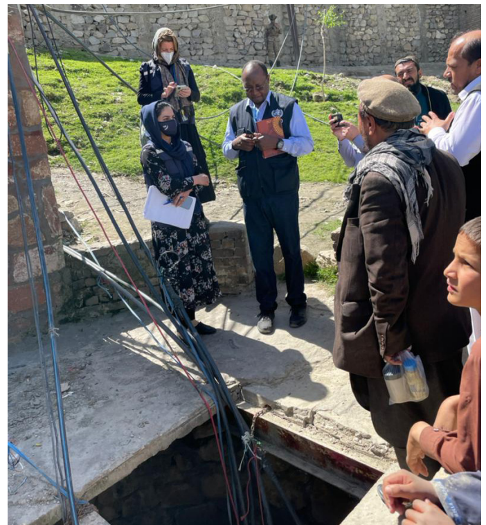
WHO and UNICEF joint investigation team inspects the contaminated water source during the AWD outbreak response in Sarobi District, Kabul Province.
