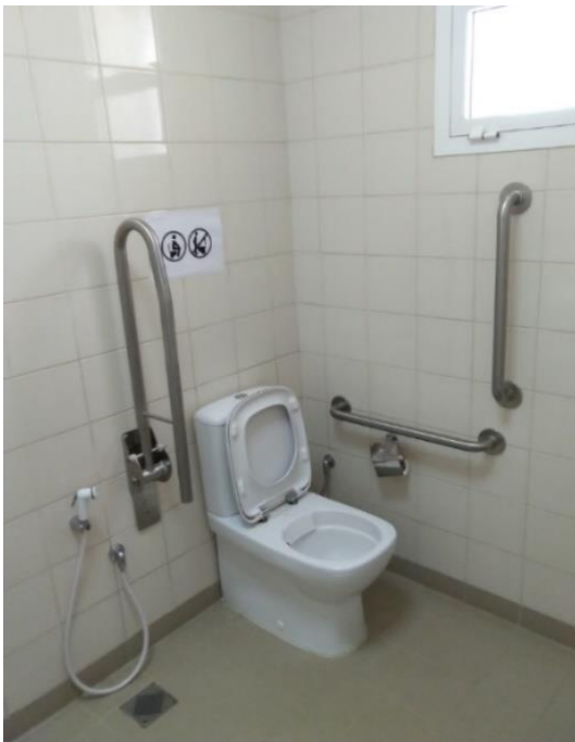
Figure 14: A toilet with accommodation for limited mobility at a healthcare facility in Oman
