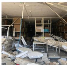
Heavily damaged central drug warehouse, WHO Lebanon
