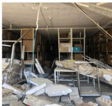
Heavily damaged central drug warehouse, WHO Lebanon
