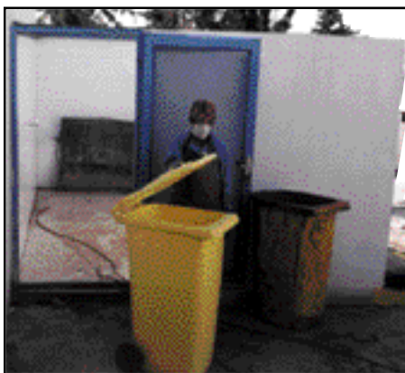
After: newly constructed room for storage of yellow bags to be incinerated (after improvement)
