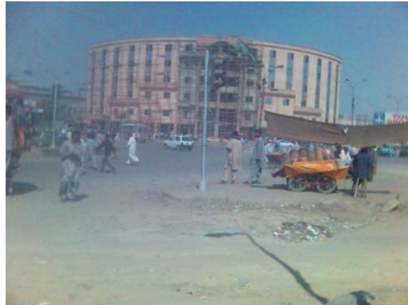
Picture-1, showing poor condition of pavement
