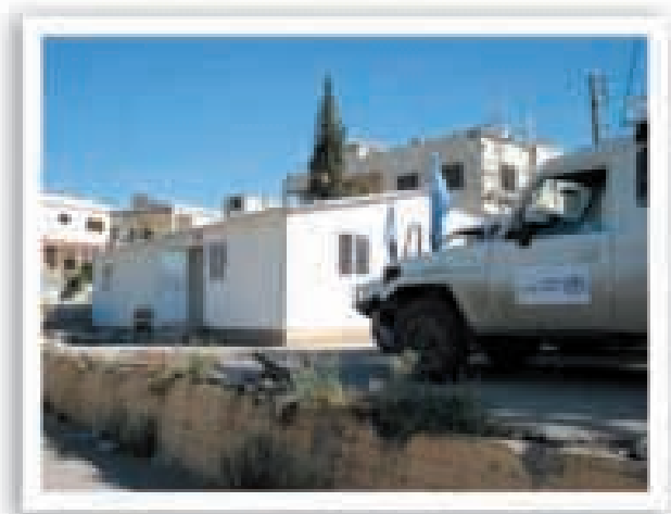
Taibeh Health Center after repair.
