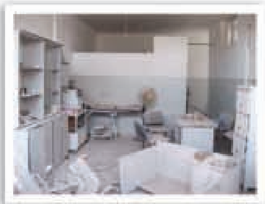
Ramieh Health Center before repair.
