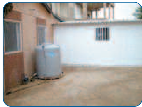
Srifa clinic after rehabilitation and installation of water tank.
