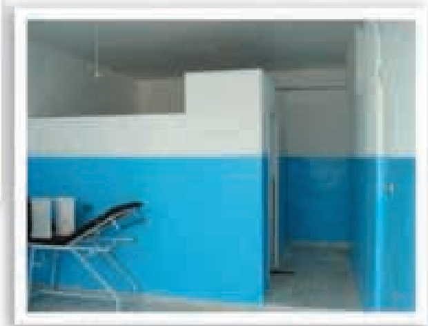
Ramieh Health Center after repair.
