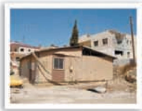
Taibeh Health Center before repair.
