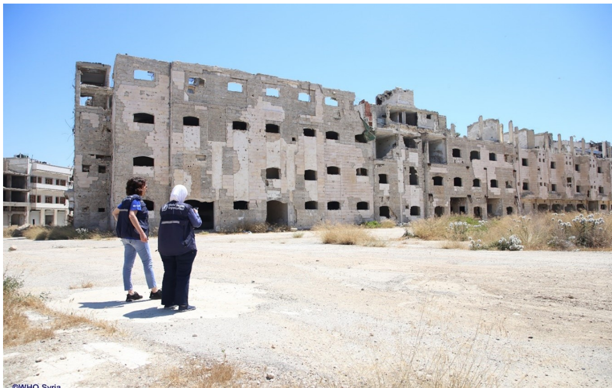
©WHO Syria Destroyed health facility in Homs governorate “Homs National Hospital”. The whole of Syria’s approach to the cholera response
